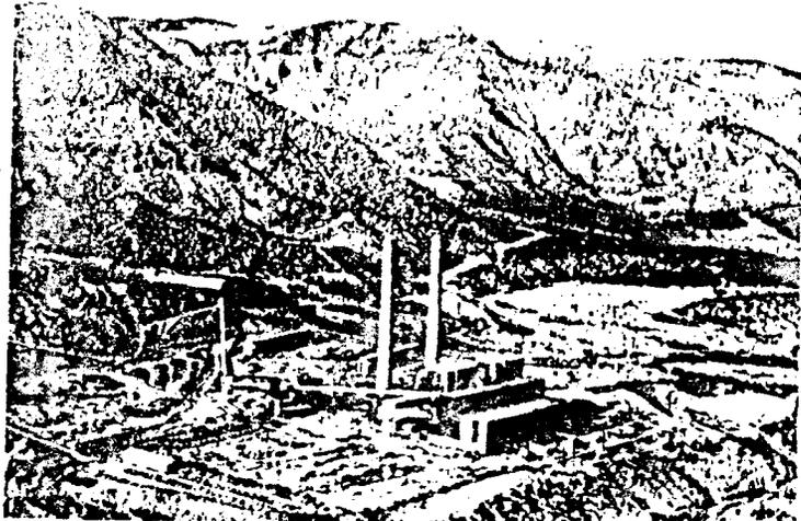
Fig. 2. The Huntington Canyon coal-fired electric generating plant of the Utah Power and Light Company. The generating capacity is 900 MW. Fuel is mined in the canyon at the left and the 345 kV switchyard is just above and to the right of the plant in this picture. It is estimated that the full electric output of a plant such as this is required to operate one 4-W electric clock per person in the United States.
